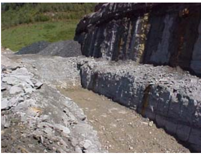
Photo shows site preparation work at Mountain Laurel.
