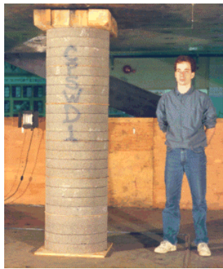
A 22" donut crib will accept approximately 550 tons of load and allow only 1.5" of convergence.
