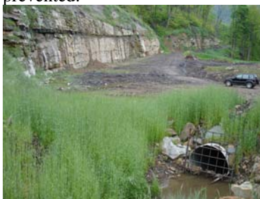
Highwall prepared for new mine opening.
